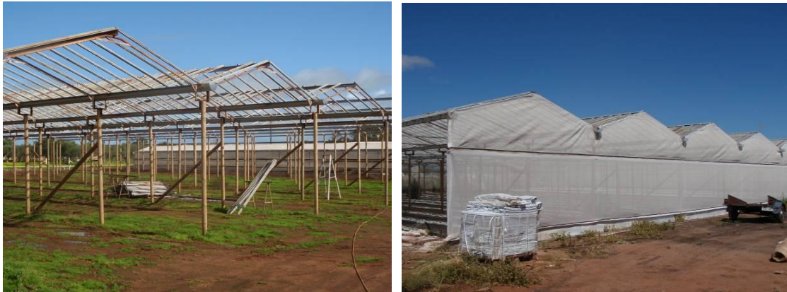
Figure 9 Construction of new greenhouse (left) and completed greenhouse (right)
